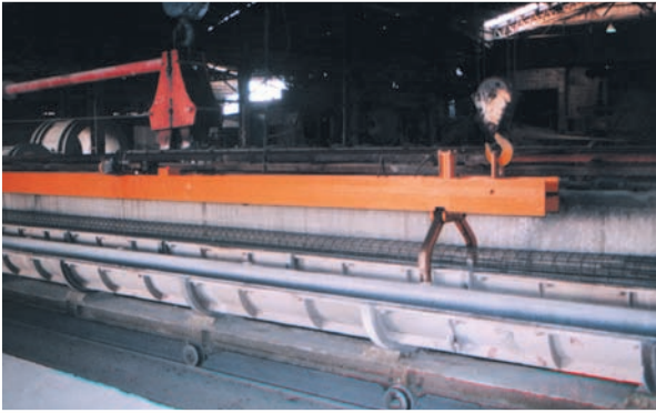
基樁投料前準備 preparation before pouring concrete of P.C. piles
